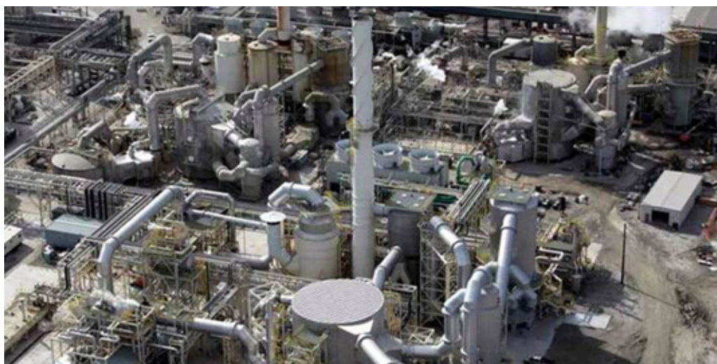
Sulfuric acid plant [DSD Chemtech]
