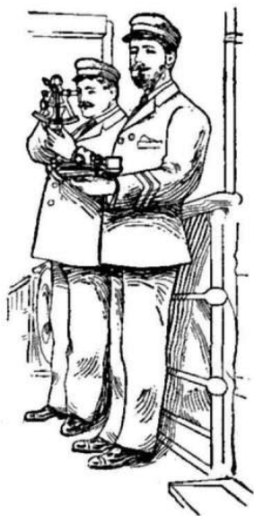
Fig. 57. Taking the altitude of the sun at sea
