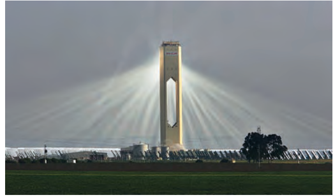
figure 11.18 At a solar thermal power plant near Seville, Spain, high temperatures are achieved by focusing sunlight from a large array of mirrors onto a boiler located at the top of the tower.
