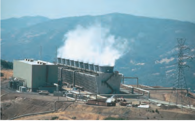
figure 11.17 The Geysers power plant in California uses geothermal energy to run steam turbines.
