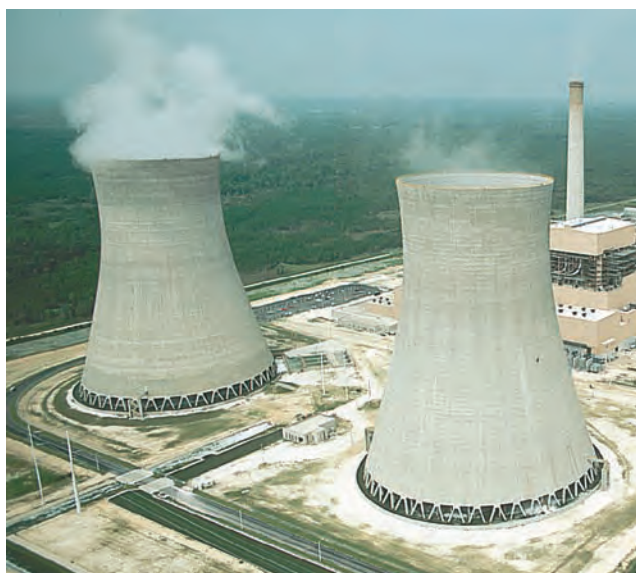
figure 11.16 The cooling towers that are a common feature of many thermal power plants transfer heat from the cooling water to the atmosphere.
